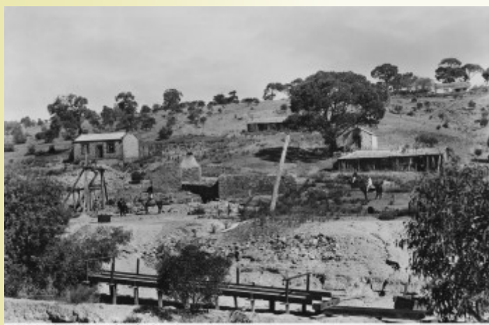
Photo above: Lady Alice mine site, approximately 1895. On the left, the manager's house and below it the poppet head of the main mine shaft. In the centre, the chimney structure is the steam house with pump. One right, front, is a wooden building, believed to be the assay office. Behind it is the small brick building that was the blacksmith's shop. The tramway lines are in the foreground, leading into the mine.
